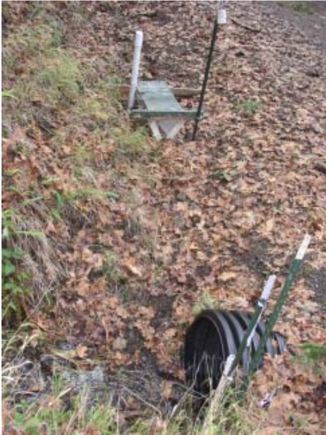
Figure 3. Pictures of Stream Crossing Culvert Installation (#1)
