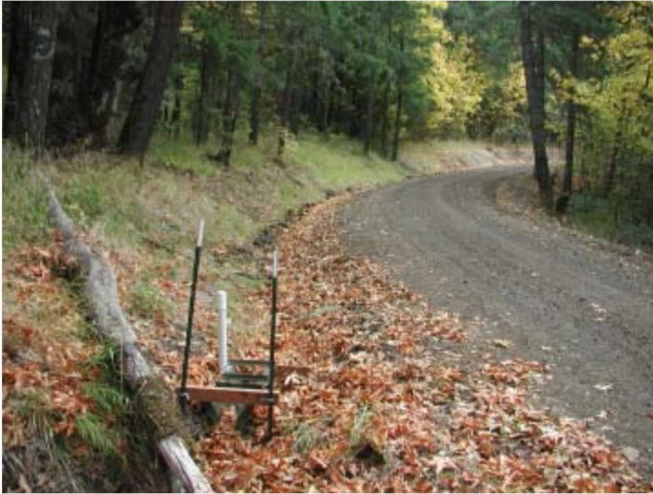
Figure 4. Pictures of Stream Crossing Culvert Installation (#2)
