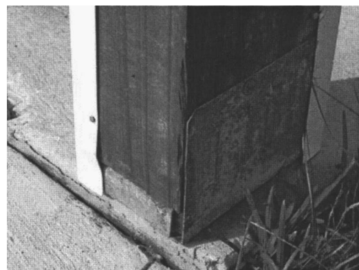
Fig. 6. Wood to concrete connection at base of porch overhang support post
