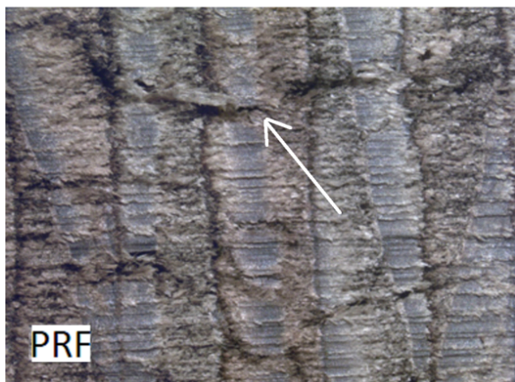
Figure 8: Crack formation in TR direction of EPI (top) and PRF (bottom) LVL due to aging.
